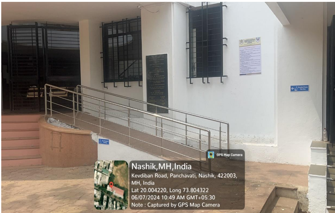
Ramp near Principal Office
